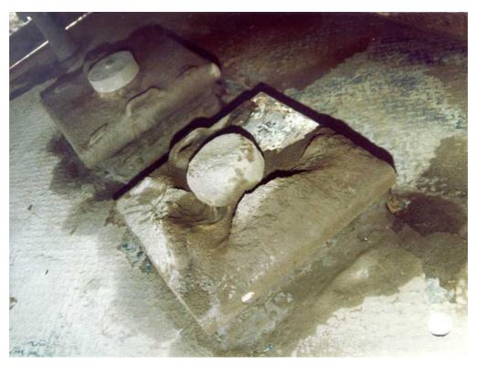
**Figure E2.** Poorly maintained PRVs. The build up of cement powder around the PRV indicates a lack of maintenance and incorrect operation. The PRV should only lift in an emergency, whereas the one pictured above appears to have been routinely lifting during delivery, resulting in the observed accumulation of powder.
