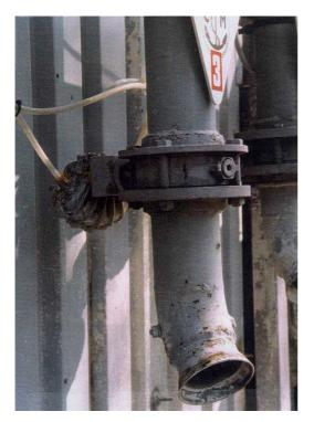
**Figure 4.** Shut-off valve located close t connection point, which is labelled.
