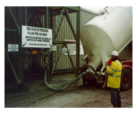
Figure 6. Delivery from tipping tanker. Note signs close to delivery point.
