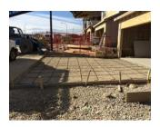
A sub-contractor was working to place concrete for a driveway. At approximately 9:00am the worker lifted the rebar at the edge along the form to allow concrete to settle underneath for proper placement within the concrete slab. The worker stated that while lifting the rebar another employee(s) had stepped on the rebar and the pressure caused the sharp end to cut his finger before he could release resulting in 7 stitches in the third finger if his right hand.
