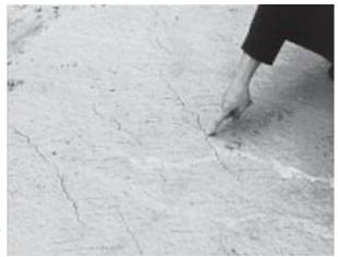
Note: Plastic shrinkage cracks should be distinguished from other early or pre-hardening cracks caused by settlement of the concrete
