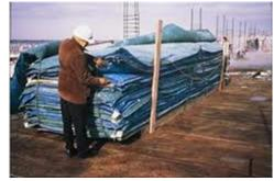
The ready-mix concrete producer and control concrete temperature and furnish concrete to comply. Concrete temperature should not exceed these values by more than 10°C. Concrete at a higher temperature requires more mixing water, has a higher rate of slump loss, and is more susceptible to cracking. Concreting in cold weather provides the opportunity for better quality, as cooler initial concrete temperature will typically result in higher ultimate strength and improved durability.
