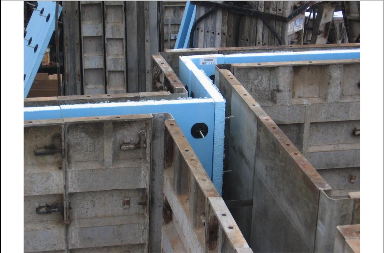
*Figure 19: Close-up view of integrally insulated wall system during forming.*
