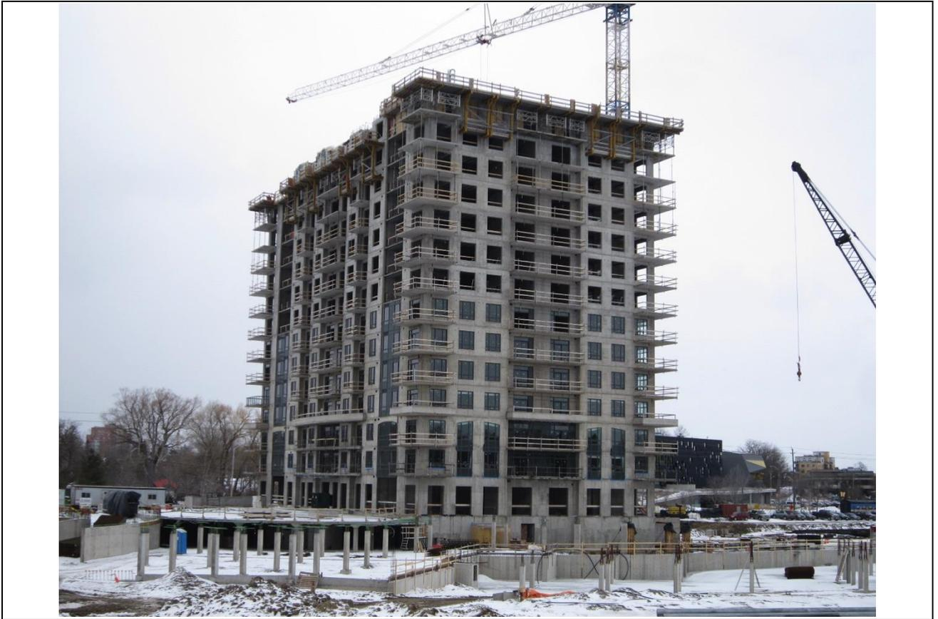
*Figure 11: Cast-in-place concrete building under construction.*
