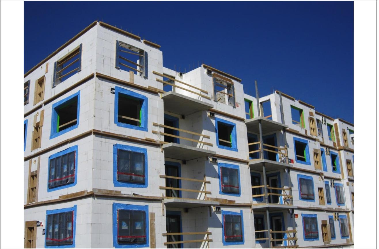
*Figure 21: ICF apartment building under construction.*
