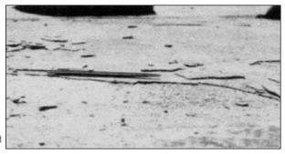
Low ambient temperature (less than about 10°C), the use of fly ash and/or chemical retarders will delay initial set of the underlying concrete and subsequently reduce the rate at which bleed water and air move upward which may tempt the finisher to apply the final finish prematurely.
